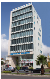
Lighthouse building Đà Nẵng
